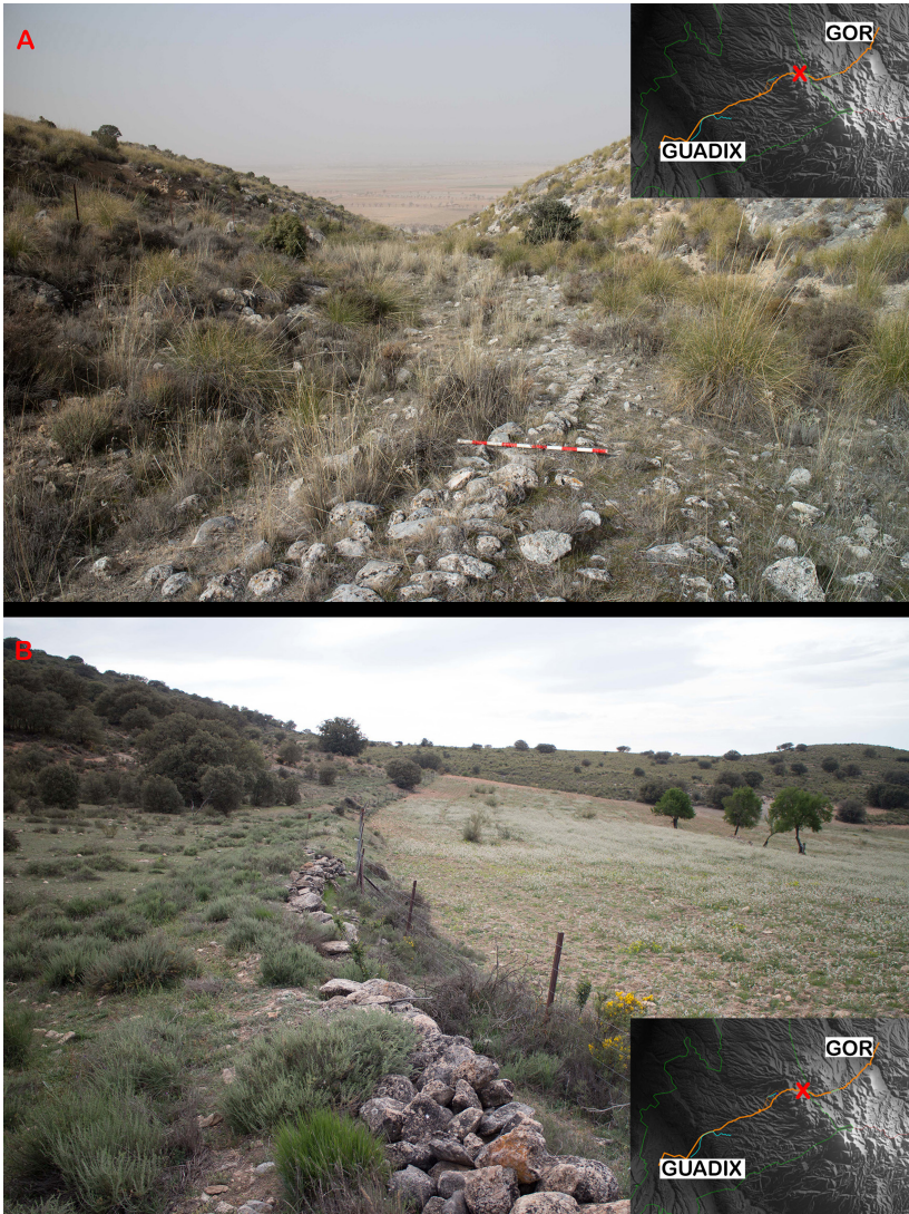
Figure 6. Paving of the road and stone-reinforced support slopes on the hillside of Cerro de Peñas Negras.
